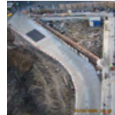
Site Layout – well planned and constructed site access roads.
