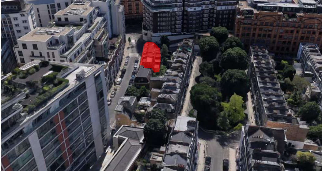
Above: Aerial view of site (highlighted red) and its surroundings prior to demolition of pre-existing dwelling houses (source Google Earth)
