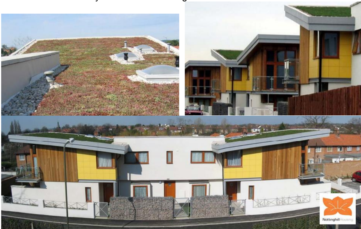
Figure 23, 24, 25: Photos of Gold Lane Social housing Project
