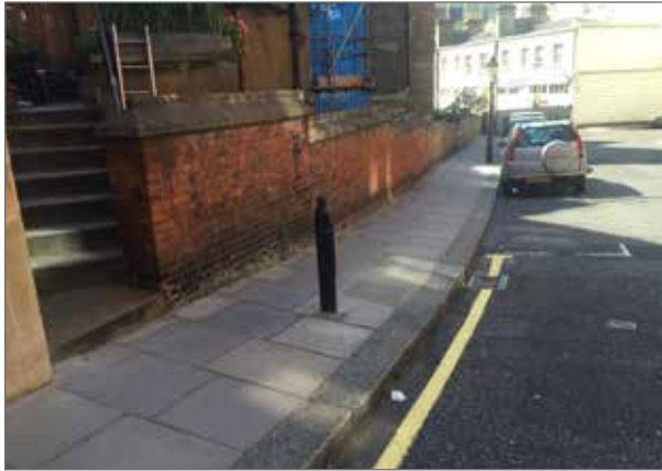
Old street light stump should be removed
